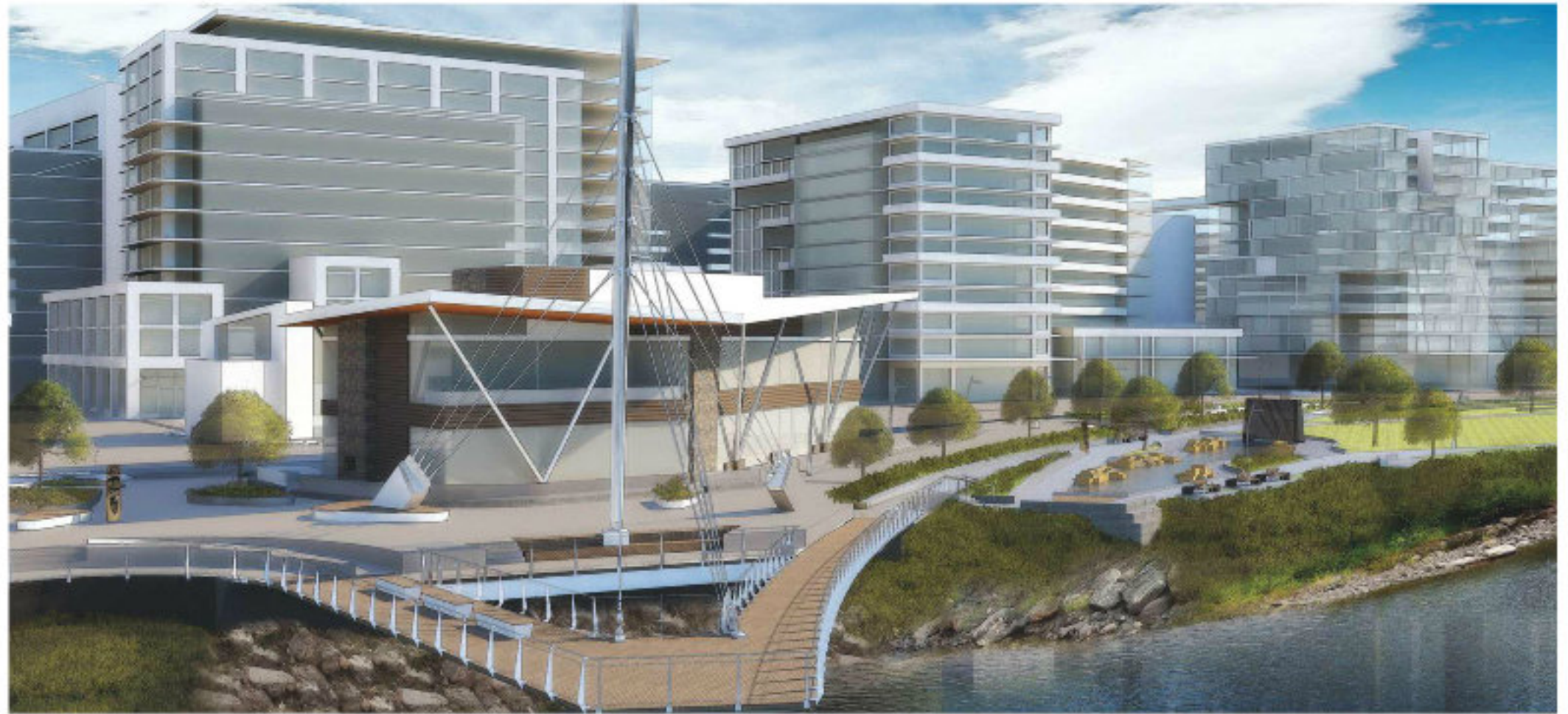
The Grant Street Pier will anchor a half-mile long waterfront park at The Waterfront Vancouver.
